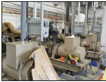
Left: the old rundown/outdated generators. Middle: the new generators being installed. Right: The generator building gets a face lift.
