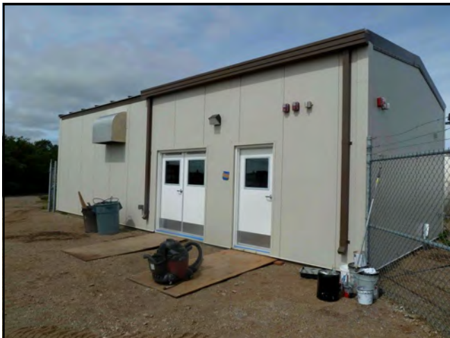
The outside of the completed generator building.
